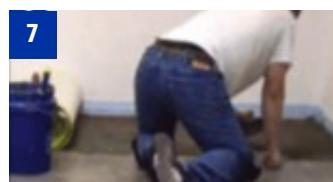
7 Key mortar into substrate with flat side of trowel, followed by mortar application with notch side.
