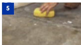
5 Wipe subfloor with a damp sponge. This will ensure good adhesion by removing dust, while dampening subfloor to help avoid moisture loss in mortar.
