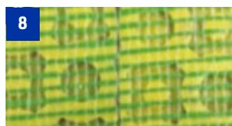
8 Decoupling Mat is installed with the **yellow** side facing upwards.
