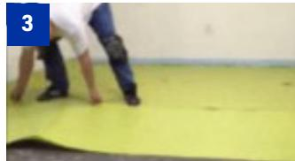
**IMPORTANT:** Maintain 1/4" spacing between mat edge and walls, columns, cabinets, etc. Pre-cut Decoupling Mat to fit using a utility knife. Dry fit into area to ensure accuracy of cuts.
