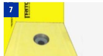
Fit Pre-Sloped Shower Pan into fresh mortar and apply pressure to ensure pan is well embedded.
